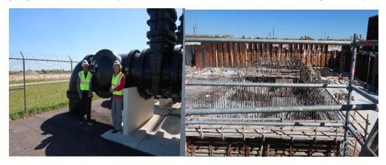
However, the scale of the reservoir is not the only reason causing a lengthy construction process. To both ensure that they settle properly and to minimize the seepage of water out of the reservoir, as part of the construction process the dirt berms that surround the reservoir must sit in place for 16 to 18 months and nothing can be done to shorten that time frame.
